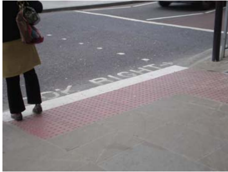
Dropped kerbs - £1000 each side or £ 2000 per crossing
