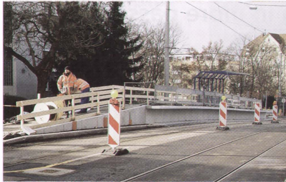
◀ Figure 1: Raised platforms constructed along one section of route U4
